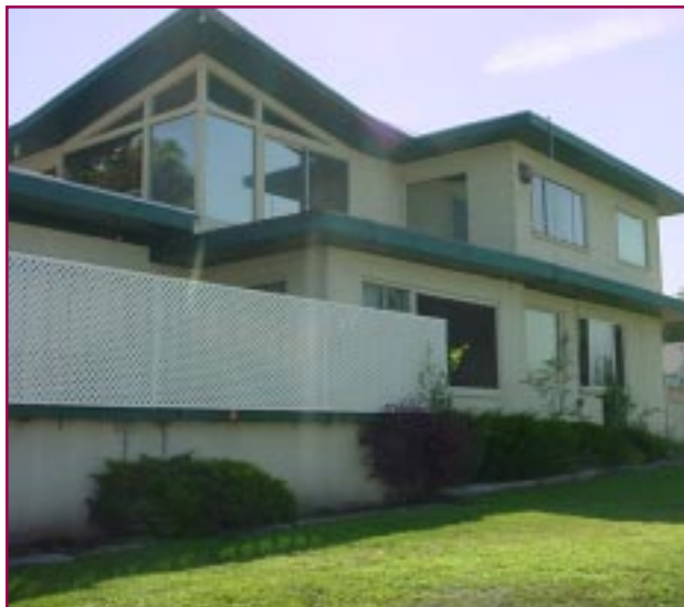
From the front the upstairs apartment for transitional housing can be seen
